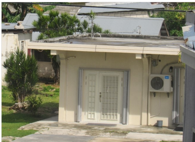
Figure 12: Home with accordion shutter door protection (shutter not deployed in this photo).
