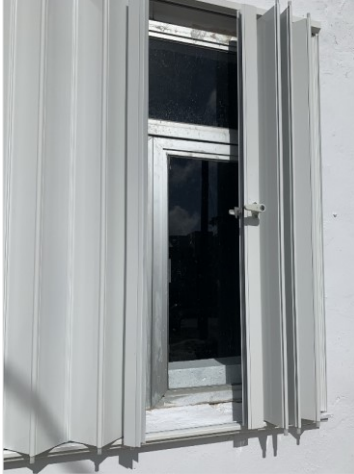
Figure 13: Residential window with typical accordion shutter with handle-style lock located in the center of the shutter.
