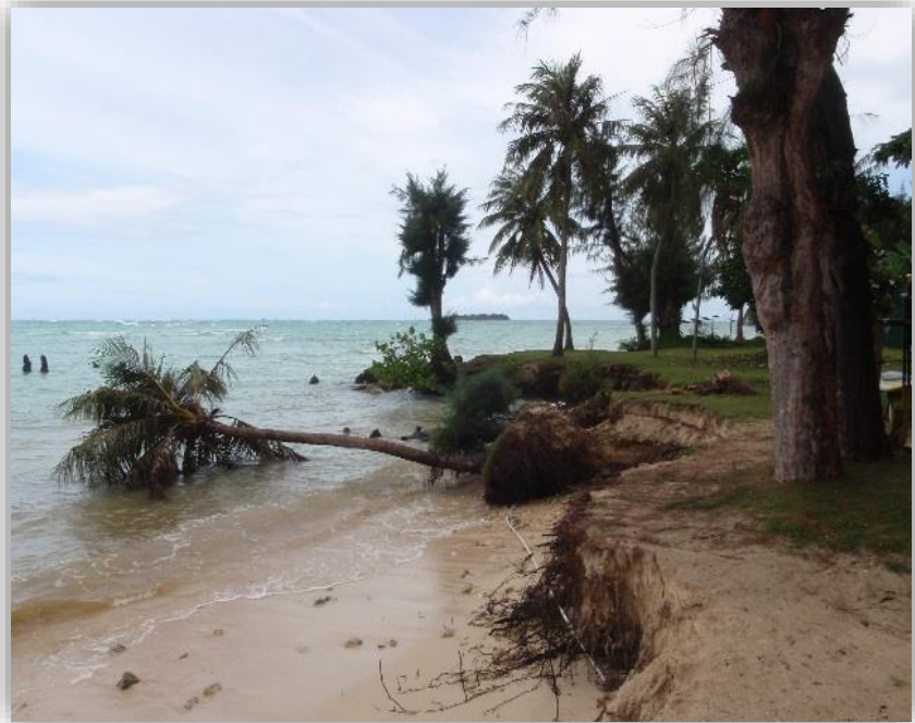
Figure 7.4 Limited vegetation types and abundance leads to eroding shoreline with utilities exposed.
