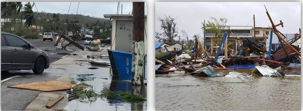
Figure 3.1 Storm-damage to the power distribution system from Super Typhoon Soudelor (left) and wreckage from Super Typhoon Yutu (right).
