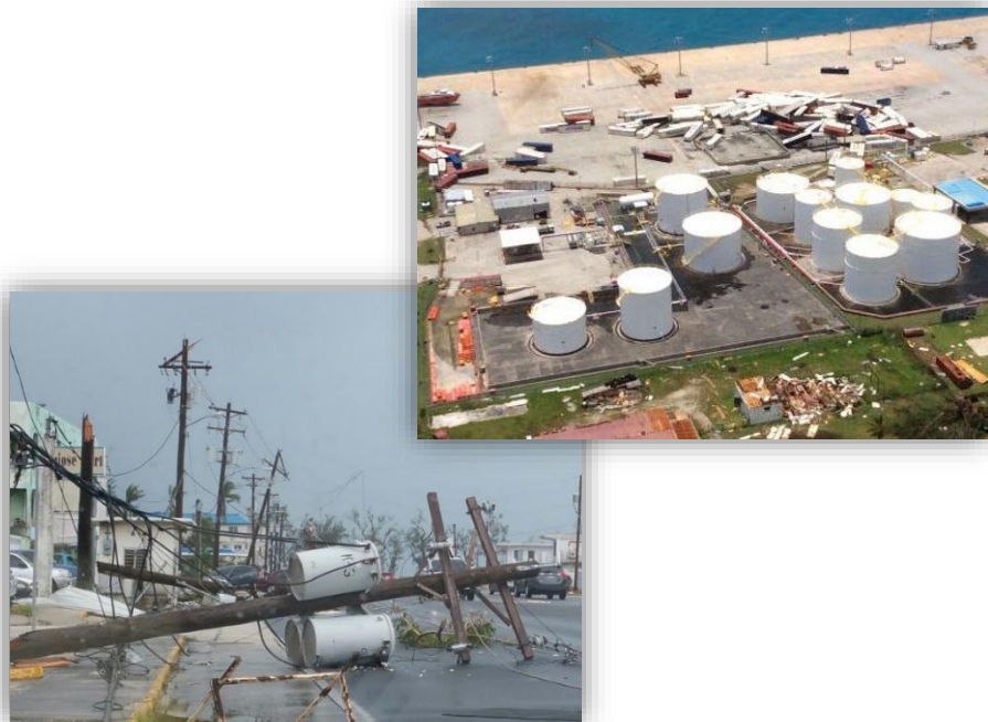
Figure 7.6 Wreckage from Super Typhoon Soudelor (August 2015). On the left are damaged utility poles and on the right is damage to the port.
