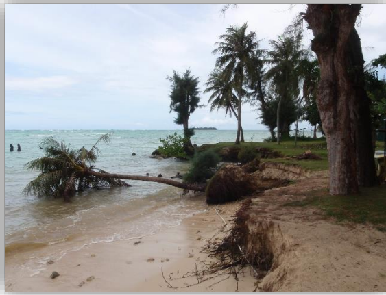
Figure E.3 Coastal erosion and sea-level rise pose challenges to the existing built environment and to future coastal development.
