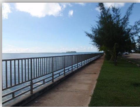
Figure E.4 Seawall protects the shoreline and provides open, recreation space.
