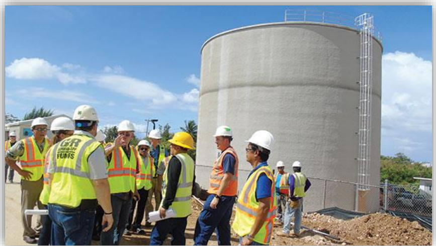
Figure 4.2 New CUC ferro-cement water storage tank will not rust.
