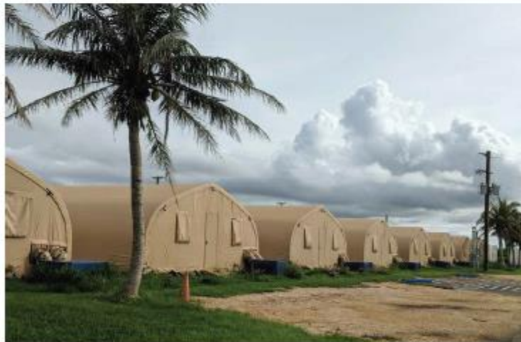
Due to extensive storm damage from Typhoon Yutu, Hopwood Middle School moved to temporary canvas tent classrooms set up on the campus of Koblerville Elementary School on Saipan. Power outages following the relocation made it difficult for students to work in extreme heat in the tent classrooms (Bautista 2019). Photo by Zena Grech, 2019.
