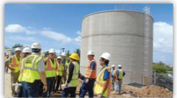
Figure 4.2 New CUC ferro-cement water storage tank will not rust.
