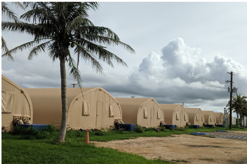
Due to extensive storm damage from Typhoon Yutu, Hopwood Middle School moved to temporary canvas tent classrooms set up on the campus of Koblerville Elementary School on Saipan. Power outages following the relocation made it difficult for students to work in extreme heat in the tent classrooms (Bautista 2019). Photo by Zena Grecni, 2019.
